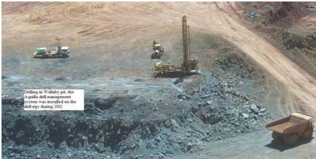
Figure 8 Drilling in Wallaby pit.
